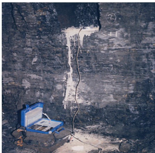
3 Monitoring of vibration in pillar of Chora 10 pit colliery
